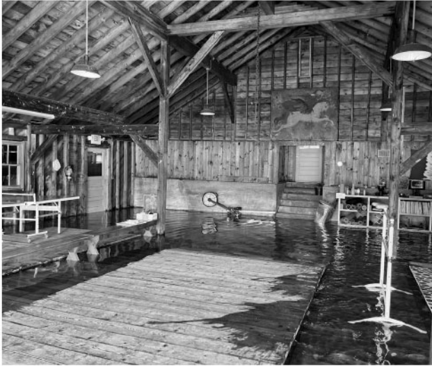
A partially submerged boathouse.
